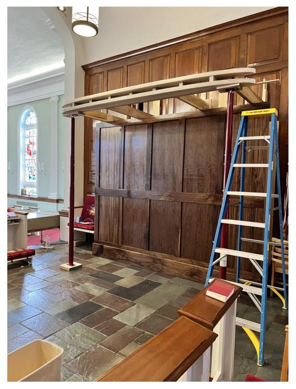
Temporary jack posts are in place so that wind chests and pipes can begin to be installed.
